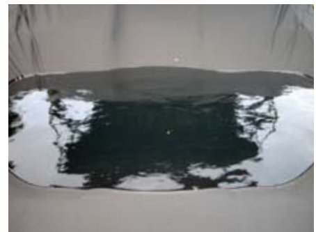
Figure 1 - 30 Gallons of water with no seepage on SurLast BW+
